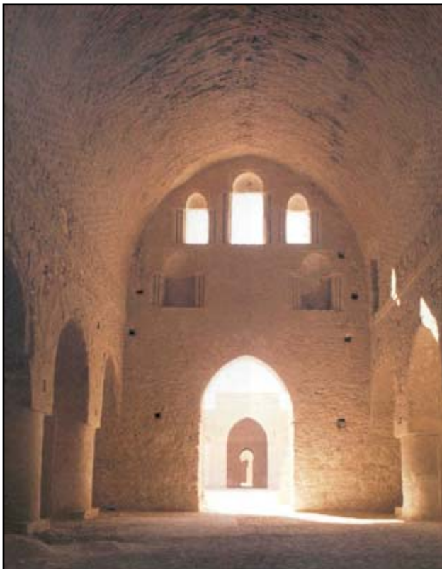
Figure 6: Ukhaidir Palace (720-800) showing the pointed arch and barrel vault of the Great Hall.
