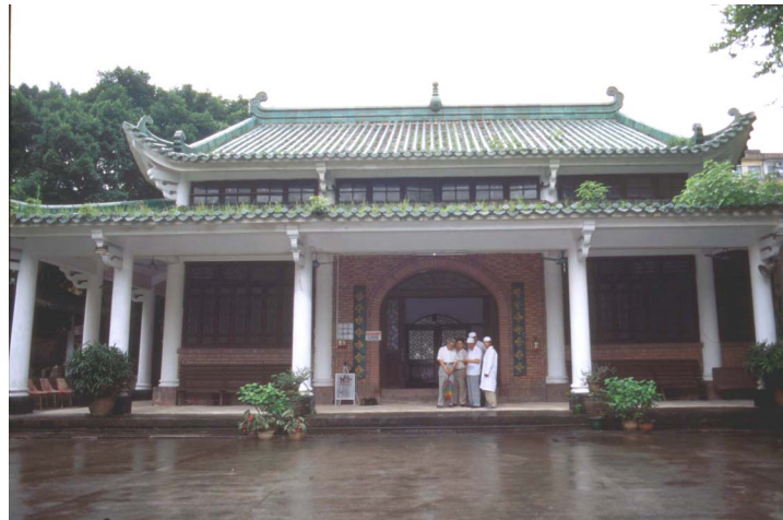
The exterior view of Prayer Hall
