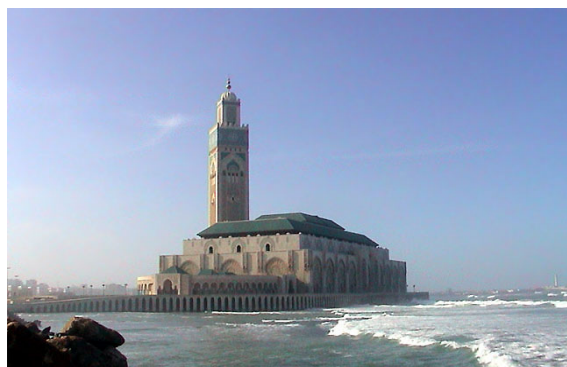
Figure 16. Exterior view of the Hassan II Mosque in Casablanca
