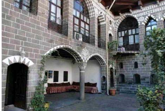
The Cahit Siki Taranci House in Diyarbakir, Turkey, is an example of a traditional courtyard-style home. Photo via Diyarbakir Association .
