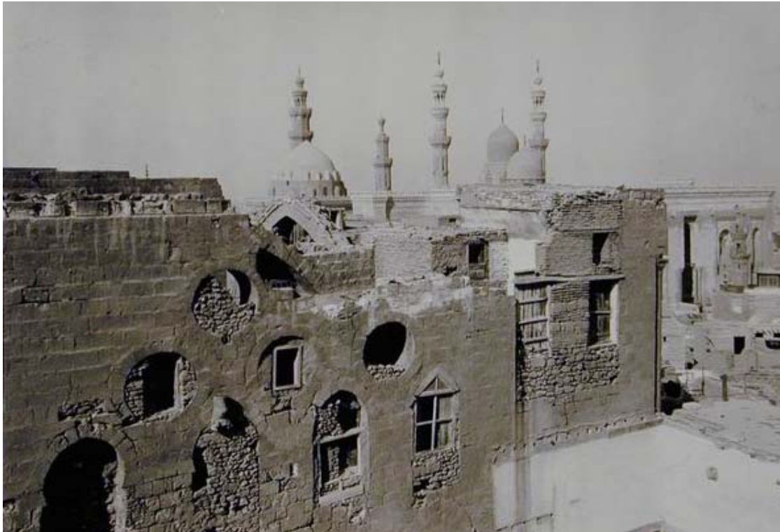
Figure 3. Northern façade of Maristān of Sultan al-Mu'ayyad Shaykh, in Cairo built in 1418-20 in the Mamluk period. Source: http://archnet.org/library/sites/one-site.tcl?site_id=2079
